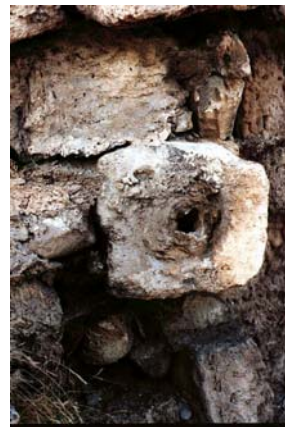
Ancient Water-pipe from Laodicea
